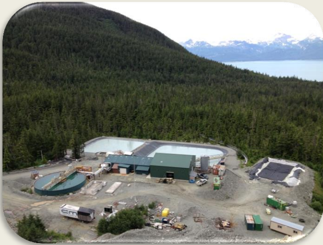
Kensington Water Treatment Plan (photo: OPMP)
