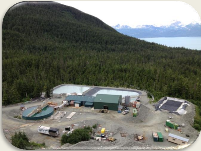
Kensington Water Treatment Facility
