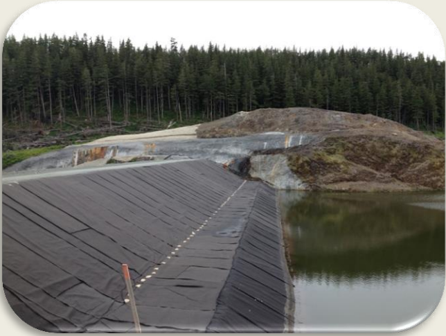
Kensington Tailings Storage Facility Dam (photo: OPMP)
