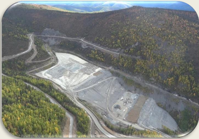
Pogo Mine Dry-Stack Tailings Storage Facility (photo: Sumitomo)
