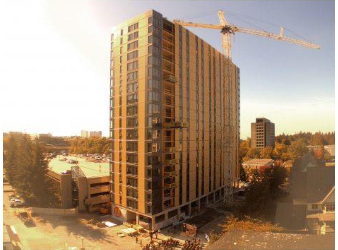
18-Story Brock Commons in Vancouver, BC Photo taken September 16, 2016.
