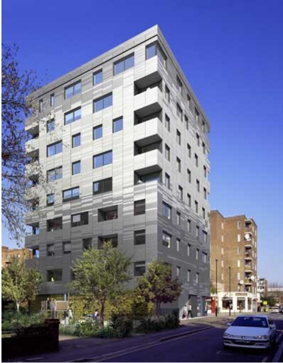
Stadthaus London, England 9-storey
