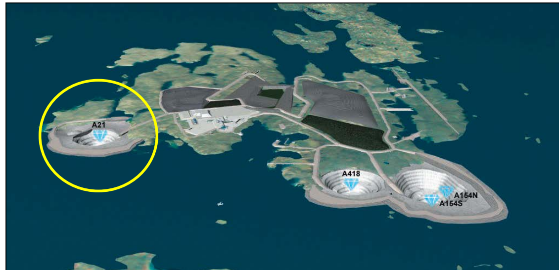
Diavik owners have approved a US$350 million investment to mine its fourth kimberlite pipe, an orebody called A21, shown at far left, using similar dike technology as shown around the A418 and A154 pipes. Courtesy Diavik Diamond Mines Inc.
