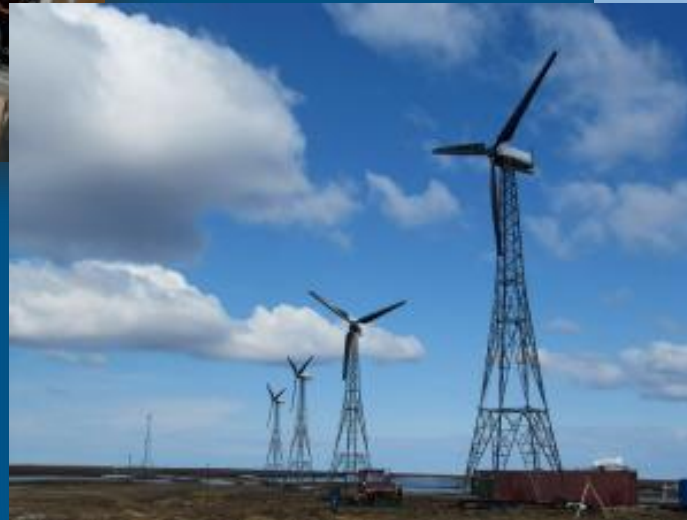
Images: Left: 20+ thermal electric stoves installed in elder and low income homes; Windmatic direct drive turbines (30-40% wind penetration annually)
